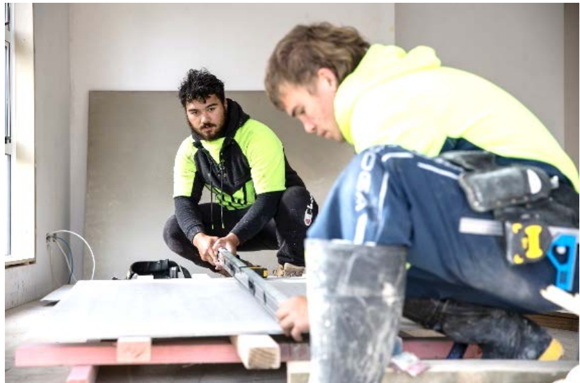
Figure 19. Qualified builder and Senior apprentice at work.
