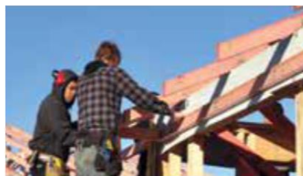
Figure 13: On-site house build
